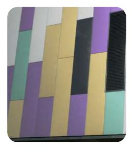
Rigid insulating core with a high thermal performance (conductivity as low as 0.0195 W/mK). Light enclosure with the possibility of mounting vertically or horizontally such. Also suitable for ceilings and partitions inner sions.
