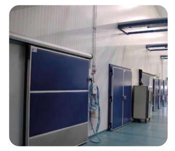
Cold Storage sandwich panel with metal faces and rigid insulating core, designed for applications that require a high degree of insulation:
